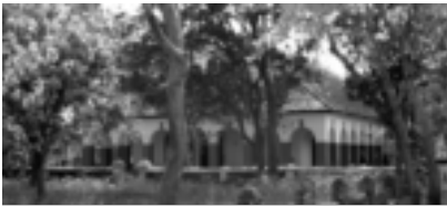
MCI church at Shantipur, near Dhamtari
